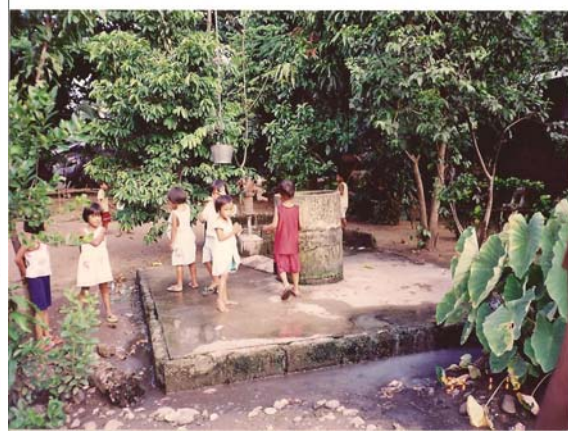
Water well system in Torrijos, Marinduque
