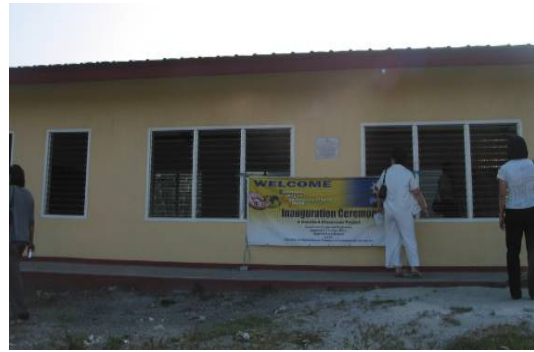
Florentino Joya Elementary School - Cavite
